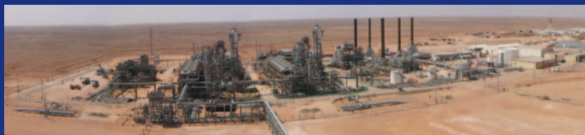
At this facility in Algeria, excess CO 2 is removed from natural gas for injection underground.
